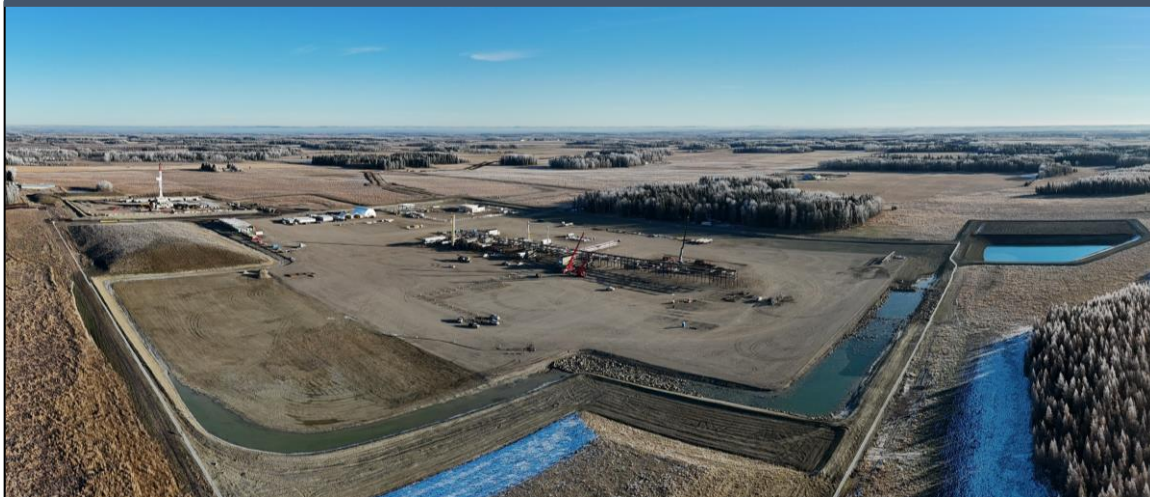
Alhambra Plant – Phase 1 Under Construction
