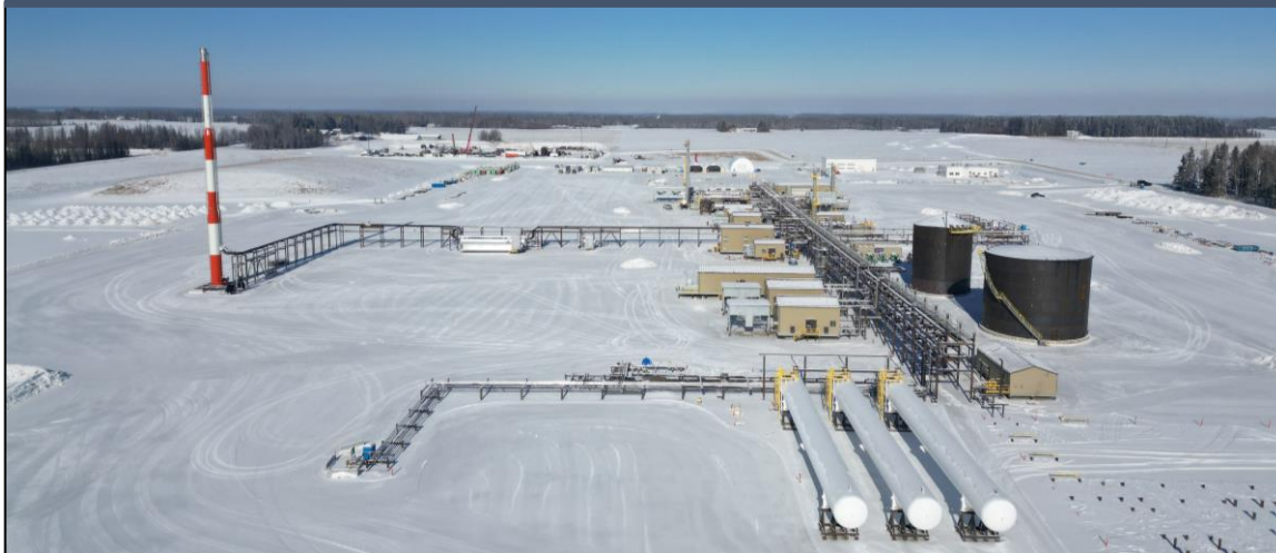
Alhambra Plant – Phase 1 Under Construction
